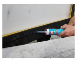
Fig. 7: Silicon spread over the gasket
