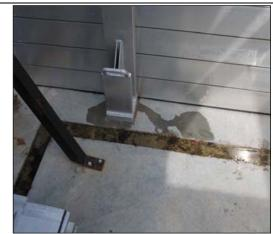
Fig. 2: Leakage at the supporting post<sup>36</sup>
