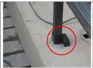
Figure 3 : Flood barrier Collad'eau-Low fastening devices
