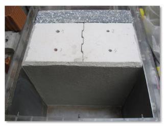
Fig. 14: Composite wall construction; single shell wall of light (aerated) concrete blocks with thermal insulation composite system.
