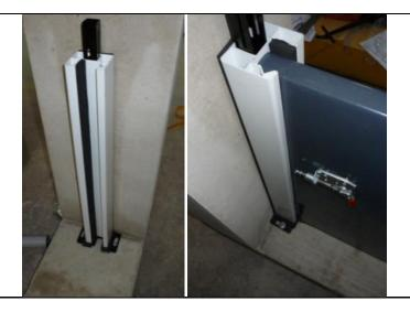
Installation of column with its steel frame and fixation with 2 anchors at the base of the steel frame, to create steel reinforced PVC column.
