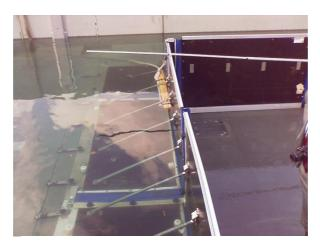
Figure 32: Aquafence – demountable perimeter flood barrier
