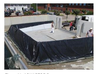
Figure 30: AQUASTOP Damm demountable perimeter flood barrier
