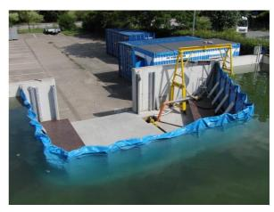
Figure 34: AquaWand system - pre-installed flood barrier
