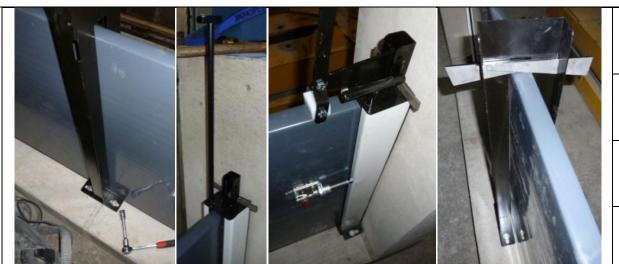
Installation of the intermediate steel frame and fixation with 4 M12 anchors in the concrete support
