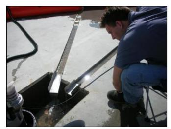
Fig. 4: Pump sump for leakage measurement <sup>3 oben3</sup>
