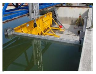
Figure 33: Spring dam system – pre-installed flood barrier
